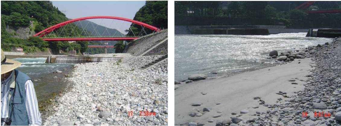
Photo 1.3 Upstream views of Kurobe River, Japan before and after sediment flushing from Dashidaira Dam and Unazuki Dam. (Photo courtesy Masaharu Fujita)
