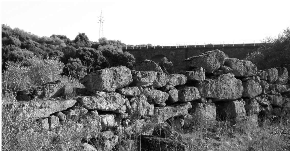
Figure 7.- The Coghinas building.
