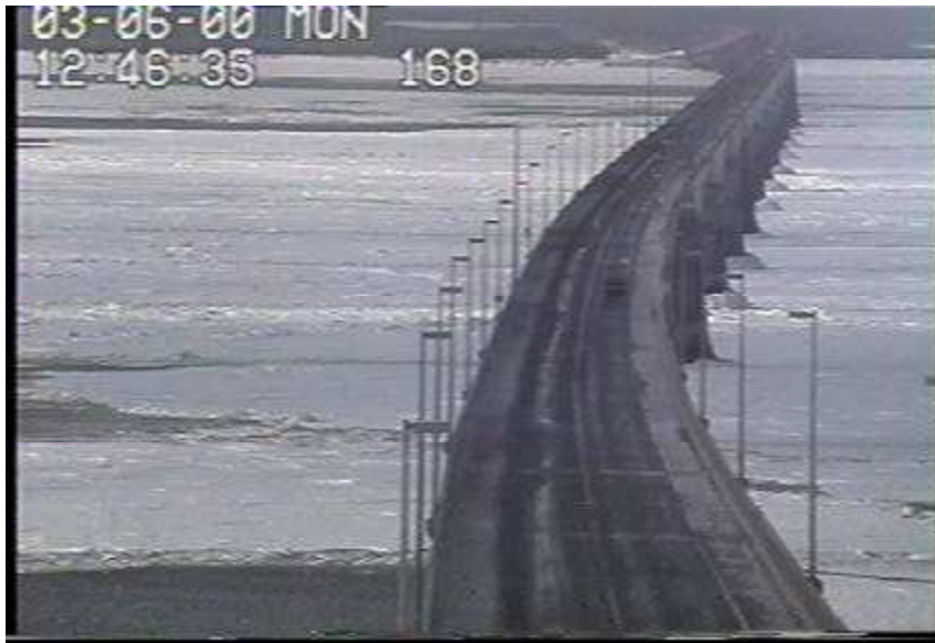
Figure 7 Ice piling on the bridge piers
