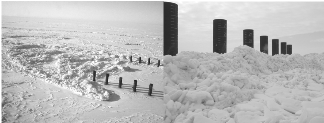
Fig.6. Two views of pile-up occurring at piles used to shelter the Sunkar drilling barge (Croasdale, 2001)
