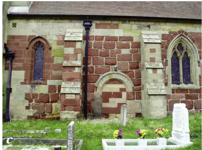
Figure 3. Arden Sandstone decay and soundness. a. heavily decayed sandstone in a church. b. sound, flaggy Arden Sandstone used in vernacular building. c. Use of any available stone in a church.
