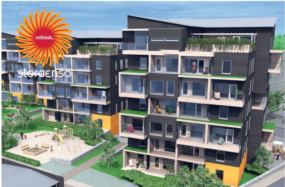
Figure 13. The Eskolantie project in Helsinki by StoraEnso utilized its modular construction with CLT technology, [63]
