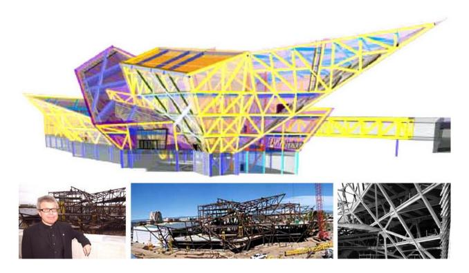
Figure 4. Art Museum in Denver (USA), Frederick S.Hemiltona building. The computer model and the construction of the building frame. Architect Daniel Libeskind. Tekla Structures software.
