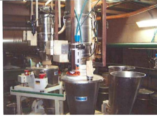
Figure 25 - - Dosing unit (Hakkarainen, 2007), P. 27
