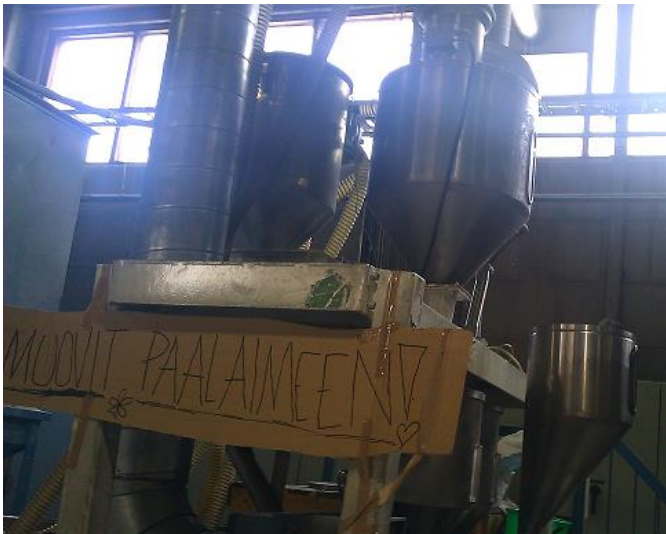
Figure 34 – Feeding hoppers in Kalliomuovi Oy.(image taken by author)
