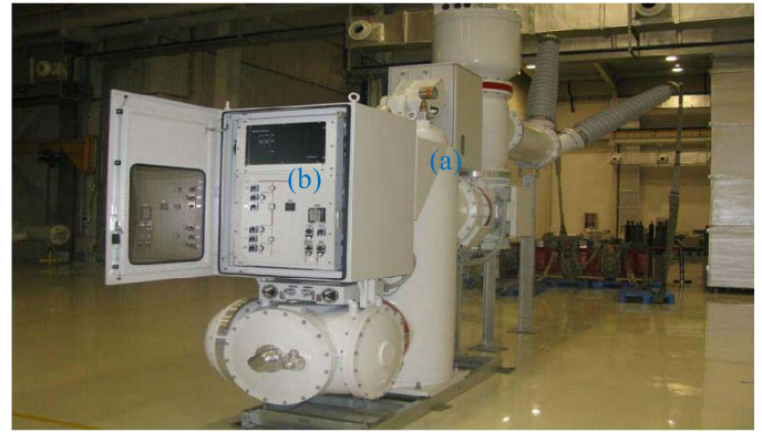
Fig. 2. Example of smart electronics close to HV devices in GIS. (a) HV GIS device. (b) Smart electronics devices.
