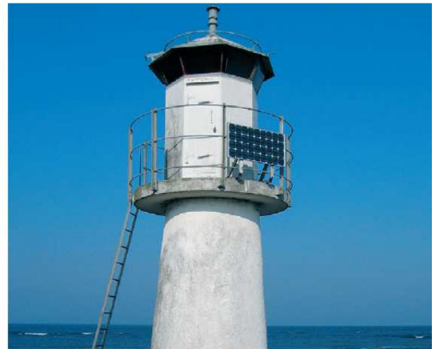
SwedModule on a lighthouse at Laus Holmar in Gotland, Sweden
