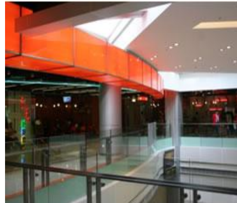
Photo 12: New glass balustrade in HTSC after renovation
