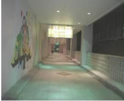
Photo9: Passageway in HTSC before renovation
