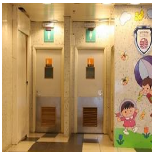
Photo 4: Washroom in FTSC before renovation
