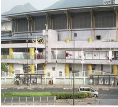
Photo 1: Outlook of FTSC before renovation
