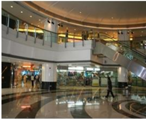
Photo 8: Passageway of LCM before renovation
