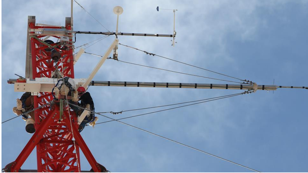
FIGURE 3.1: Picture of the M4 tower with instrumentation boom reproduced from Clifton [30].
