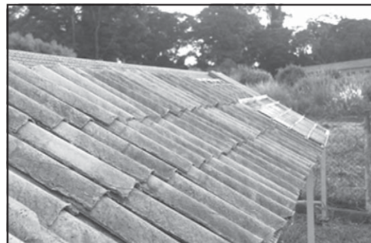
Figure 4 – Metallic structure for weather exposition of roofing elements.
