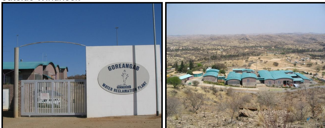
Figure. 13 and 14: The New Goreangab Water Reclamation Plant just outside Windhoek
