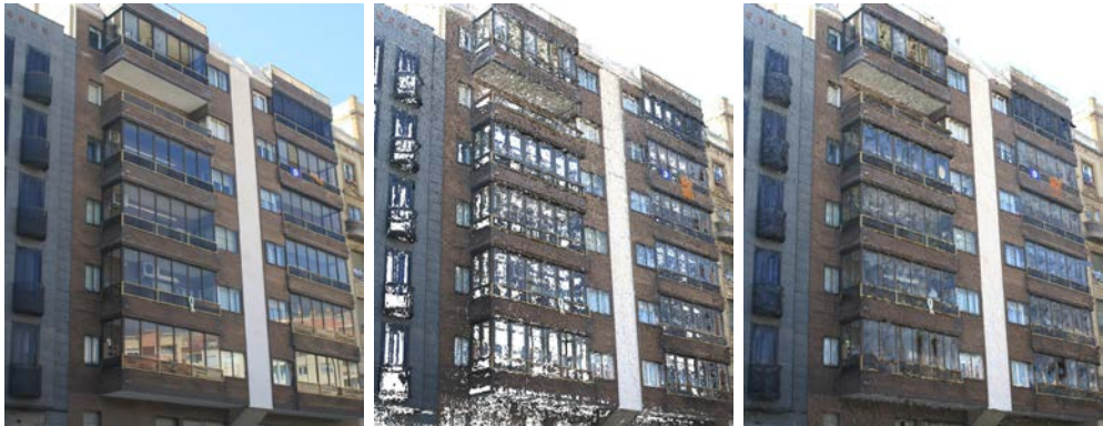
Figure 5.3: Glass window behavior goes from nearly refractive to nearly mirror-like depending on incident angle and glass treatment (e.g. reflective films). In this reconstruction example (Colmap), window panes appear noisy and sparse, and the resulting mesh has significant noise.
