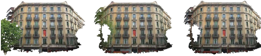
Figure 5.23: Impact of the semantic segmentation mask for weighting pixel contributions. From left to right: (1) Reconstructed model (Colmap) with per-vertex color. Color pollution on the facade near the tree is hardly visible. (2) The output of our pipeline but disabling pixel-weighting when generating the texture. Overall color reproduction is much better but the left side of the facade has serious color artifacts. (3) The output of our complete pipeline; despite trees were not reconstructed, tree pixel colors do not contribute to the facade.
