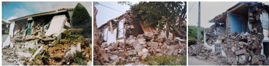
357 Figure 5. Examples of evaluated buildings belonging to each damage grade from the EMS-98 scale
