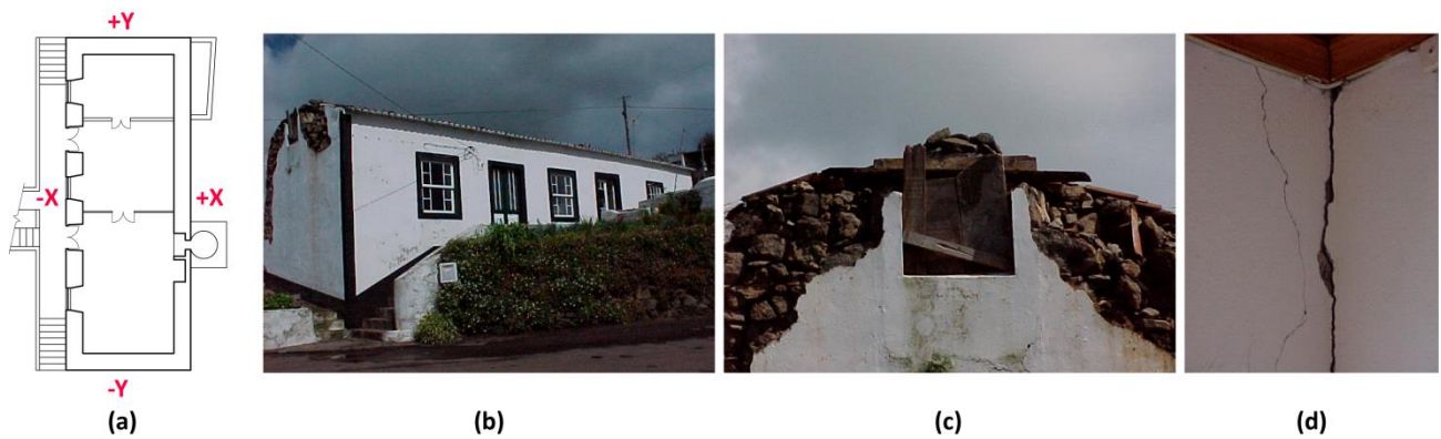
630 Figure 18. (a) Building plan and directions nomenclature; (b) main façade of the building; (c) collapsed gable 631 wall; and (d) visible damage at the wall-to-wall connections from the interior of the building
