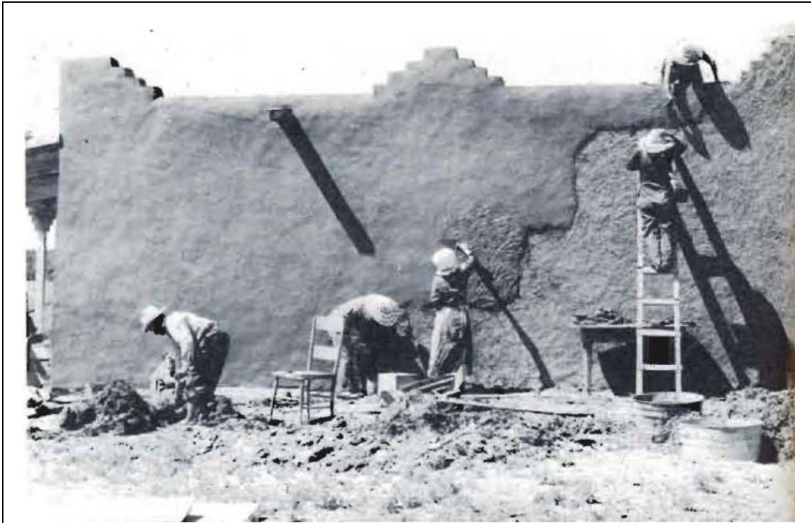
Figure 30. Coating of an earth house with mud, near Santa Fe, New Mexico, ca. 1930. Photograph by Russell Lee, Library of Congress.
