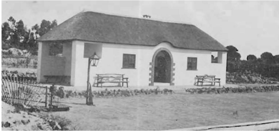
Figure 60. Wayside station constructed of pisé, Simondium, South Africa, designed by Mr. Herbert Baker. Built 1919. Photograph from Cottage Building in Cob, Pisé, Chalk & Clay, page 23.
