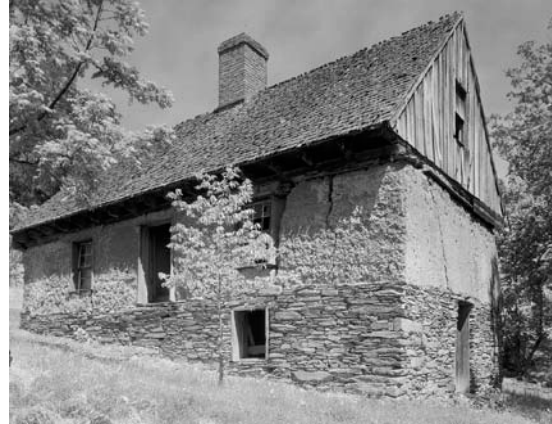
Figure 3. Rammed earth slave quarters at Bremono Recess, Fork Union vicinity, Fluvanna County, Virginia. Built in 1815 by General John Hartwell Cocke. The HABS database cites this building as adobe not rammed earth. Photograph from Library of Congress, Prints & Photographs Division, LC-DIG-csas-04761.
