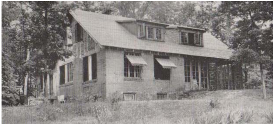
Figure 77. R. C. Cook Residence, Lantham, Maryland, 1929. To keep costs to a minimum, Cook used rammed earth construction techniques uniquely. Photograph from The Rammed-Earth House by Anthony Merrill, illustration insert.
