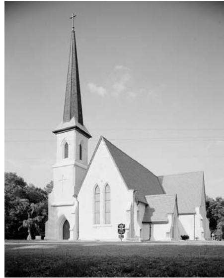
Figure 4. Church of the Holy Cross, Stateburg vicinity, near Sumter, South Carolina. Completed in 1851, the congregation agreed to the rammed earth building technique only because of its low cost. Photograph from Library of Congress, Prints & Photographs Division, HABS SC,43-STATBU.V,1--20.
