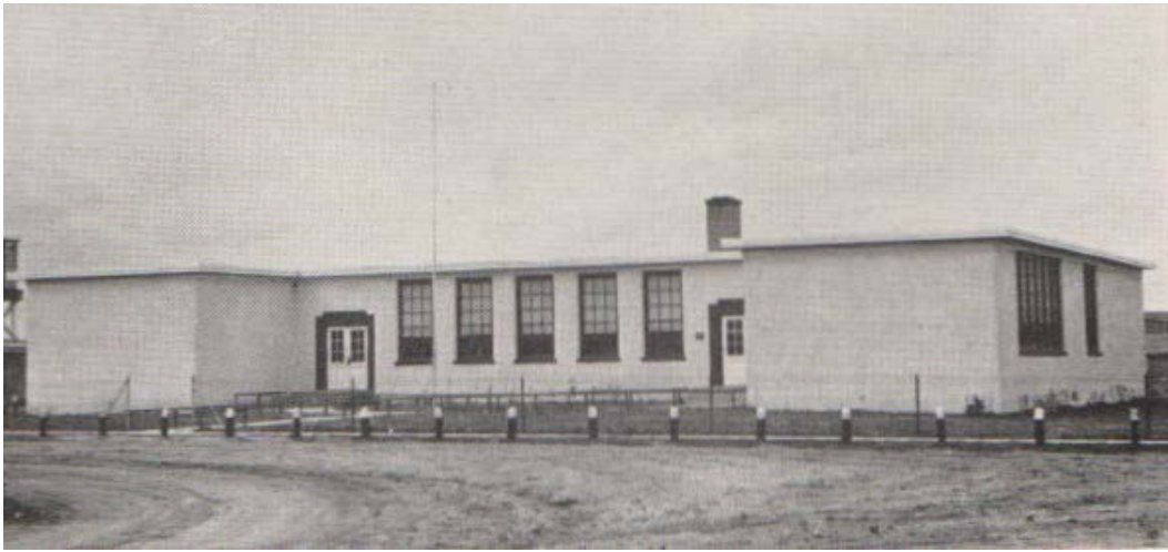
Figure 81. Indian School constructed of rammed earth by Elbert Hubbell in Wanblee, South Dakota in 1938. Photograph from The Rammed-Earth House by Anthony Merrill, illustration insert.
