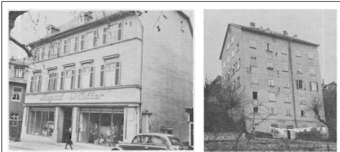
Figure 49. Two rammed earth buildings in Weilburg, Germany designed by Wilhem Jacob Wimpf. A home constructed ca. 1820 with a post-World War I commercial storefront conversion on the first floor (left) and a seven-story apartment complex constructed in 1828 (right) was renovated in 1978. Photographs by Lydia A. and David J. Miller, 1949 from manuscript of Manual for Building a Rammed Earth Wall, page 50. University of Northern Colorado archives.
