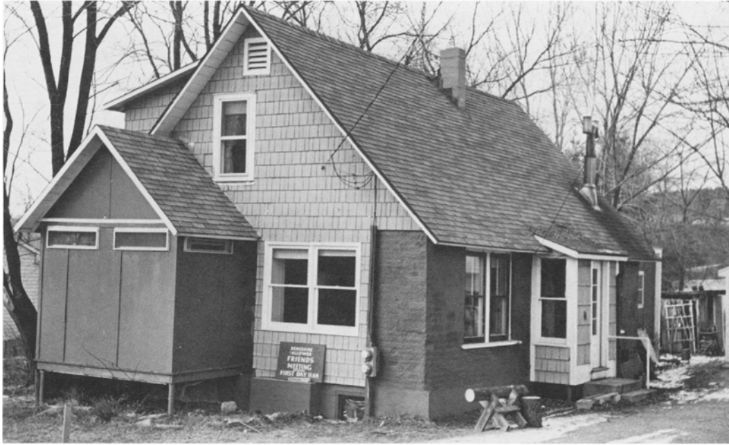
Figure 89. Lester and Margaret Clarke's Home in the Bershire Hills of western Massachusetts, 1951. Documented in 1983, it had survived thirty-one harsh northeastern winters without failing. Photograph from Bulletin of the Association for Preservation Technology article "A Rammed Earth House in Massachusetts," page 35. Photograph 1983.
