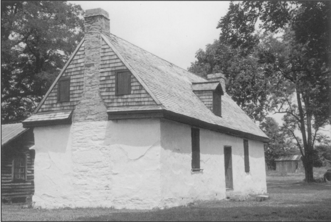
Figure 67. Overseer’s quarters at Pea Hill Plantation, Brunswick County, Virginia, ca. 1820. Lime-based roughcast or lime-based stucco was used as the finish for rammed earth buildings constructed during the nineteenth century in Virginia. 183 Photograph reprinted from “Pisé Construction in Early Nineteenth-Century Virginia” by Gardiner Hallock, Perspectives in Vernacular Architecture 11 (2004), page 46. Attributed to the Virginia Department of Historic Resources.
