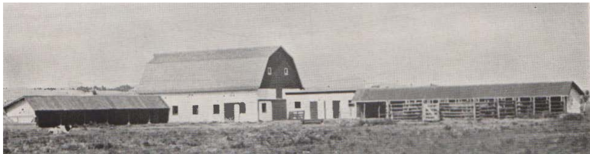
Figure 80. A massive rammed earth barn built on the Pine Ridge Indian Reservation in South Dakota ca. 1935 by Elbert Hubbell. Photograph from The Rammed-Earth House by Anthony Merrill, illustration insert.
