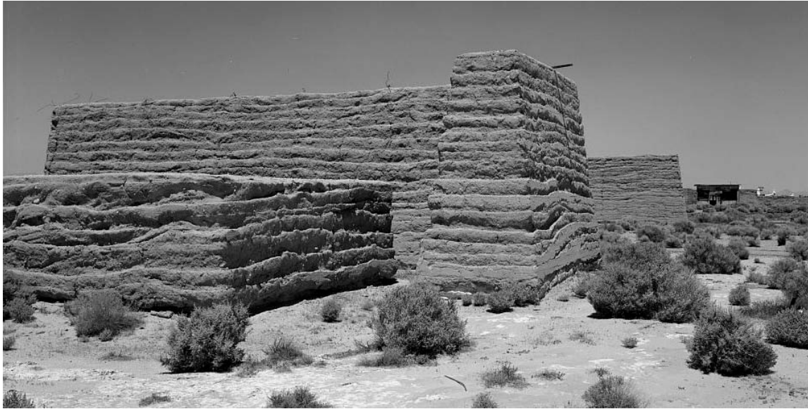
Figure 85. Perspective view of AR-8, a bomber revetment at Edwards Air Force Base near Kern, California built in 1943. Photograph from Library of Congress, Prints & Photographs Division, HAER CA-308-B-5.
