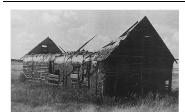
Figure 99. The remains of a rammed-earth farmhouse near Fairfield, North Dakota. Photograph from “German-Russian Houses in Western North Dakota” by Alvar W. Carlson, page 52.
