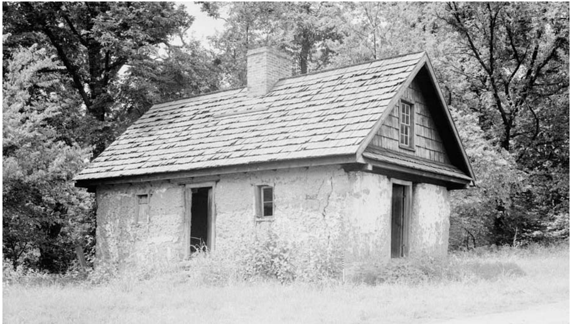
Figure 65. Slave quarters at Bremo Plantation, Fluvanna County, Virginia, ca. 1820. The flared eaves, seen on the gable end, were designed to protect the rammed earth walls by diverting rainwater away from the structure. 173 Photograph from Library of Congress, Prints & Photographs Division, HABS VA, 33-FORKU.V,1--22.
