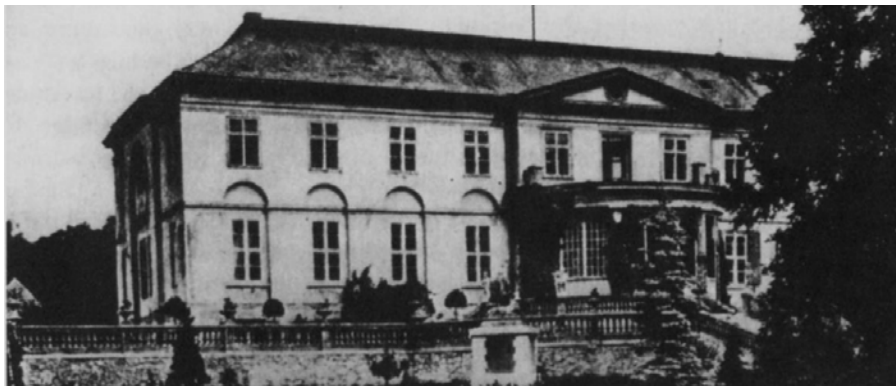
Figure 47. Palace Kleinmachnow, near Zehlendorf outside of Berlin, Germany, 1798. Photograph reprinted from “François Cointereaux's École d'Architecture Rurale (1790-91) and its Influence in Europe and the Colonies,” by Louis Cellauro and Gilbert Richaud, page 133.
