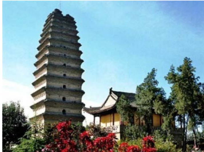
Figure 39. The Small Wild Goose Pagoda in Xi'an, Shaanxi, China is built of rammed earth walls with set-in brick pillars. It was originally constructed between 707 and 709 AD. Photograph from "Research on 3D Reality-based Modeling and Virtual Exhibition for Cultural Sites -Taking the Small Wild Goose Pagoda in Tang-Dynasty as the Case" by Jun Liu and Guo-hua Geng, page 307.
