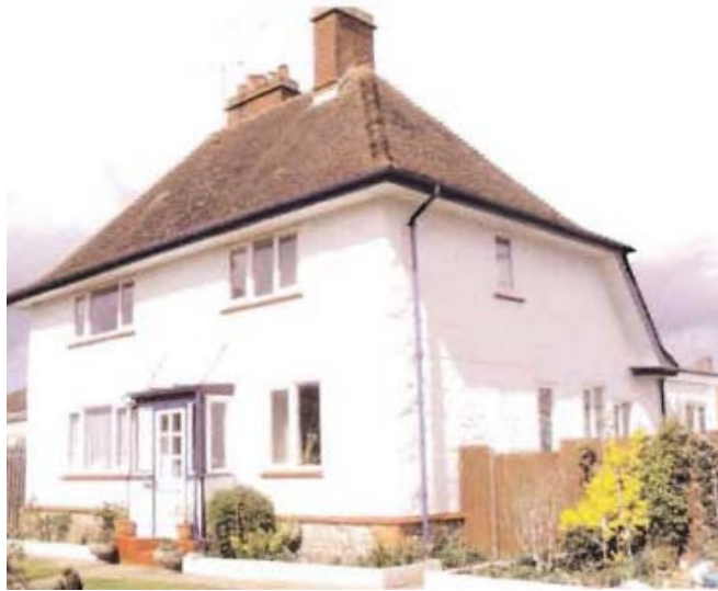
Figure 62. Rammed chalk house in Amesbury, Wiltshire, United Kingdom built ca. 1920. Photograph from Rammed Earth; Design and construction guidelines, page 5. The photo is credited to Peter Walker.
