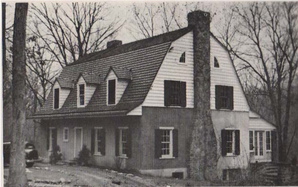
Figure 76. The Humphrey House, Washington, D.C., 1924. Merrill notes that the first floor rammed earth walls must hold up the timber second floor, attic space, and massive tile roof. Photograph from The Rammed-Earth House by Anthony Merrill, illustration insert.
