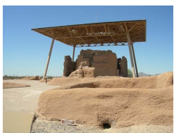
Figure 2. Casa Grande rammed earth structure at Casa Grande Ruins National Monument, Coolidge, Arizona, built ca. 1350. Photograph by the author, 2009.
