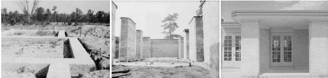
Figure 78. Rammed earth construction in-process photographs for Gardendale. Thomas Hibben and Arthur Rothstein, Photographers, 1937. Photographs from Library of Congress: LC-USF347-015512-C, LC-USF347-015511-C, and LC-USF34-025290-D.
