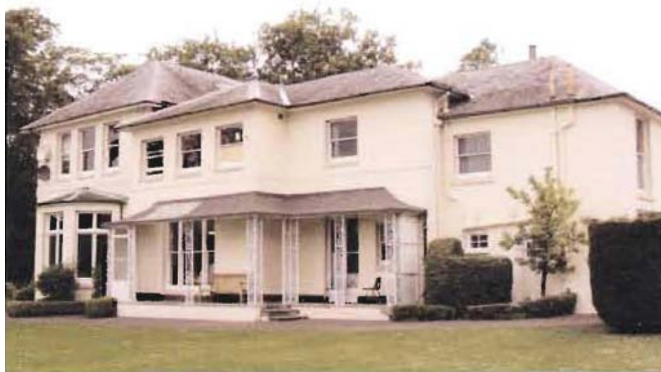
Figure 54. Five-story Victorian rammed chalk houses in Winchester, Hampshire (top) and a rammed chalk country house in Andover, Hampshire (bottom) constructed ca. 1840. Photographs from Rammed Earth; Design and construction guidelines and credited to Peter Walker, page 5.
