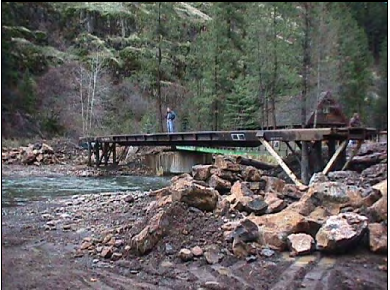
Figure J: 1997 Flood damage on Mill Creek (University of Oregon, Community Planning Workshop)
