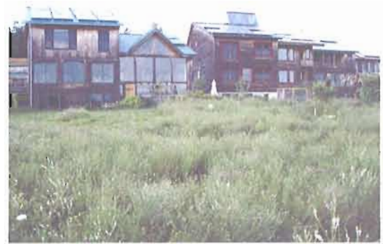
Figure 14. Passive solar, solar hot water, and solar photovoltaics (PVs) in SONG. Photo by author.
