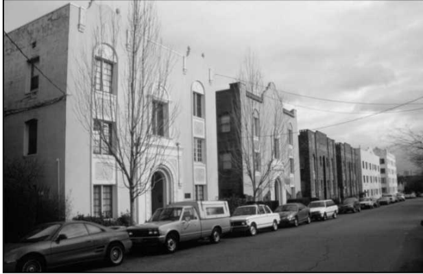
1920s apartment buildings on one of the most intensively developed blocks in the Nob Hill area
