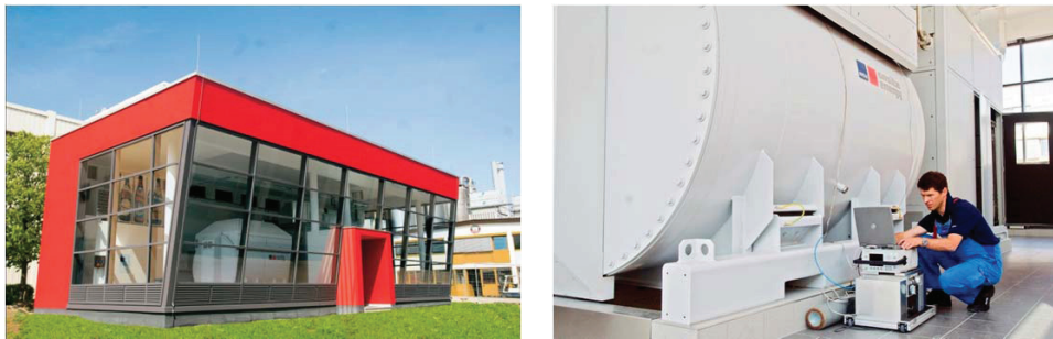
Figure 9: HotModule fuel cell HM300 at Germany's largest private brewery Erdinger Weißbräu.
