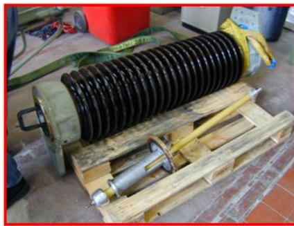
Remove connecting rod of Pole A
