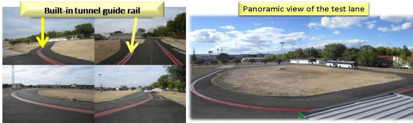
Figure 2. Partial and panoramic views of the test circuit (385 m. long).
