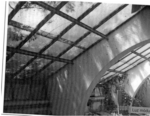
Figure 11: The attachment of the mullions on the arches at bay 1
