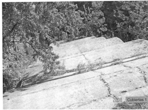
Figure 7: External aspect of the vaults
