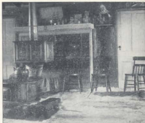
Typical Old-Time Newfoundland Kitchen.
