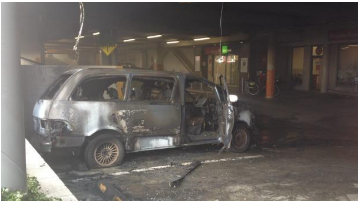
Figure 11-1: Burnt van inside a shopping mall parking in Auckland, New Zealand (Retrieved from stuff.co.nz [4])
