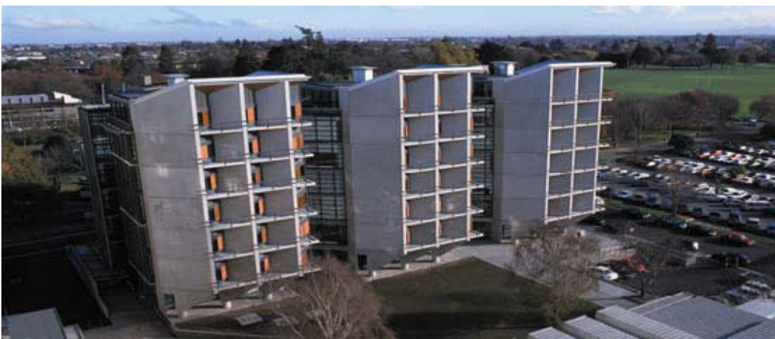
Figure 6-2: Erskine building at the University of Canterbury.
