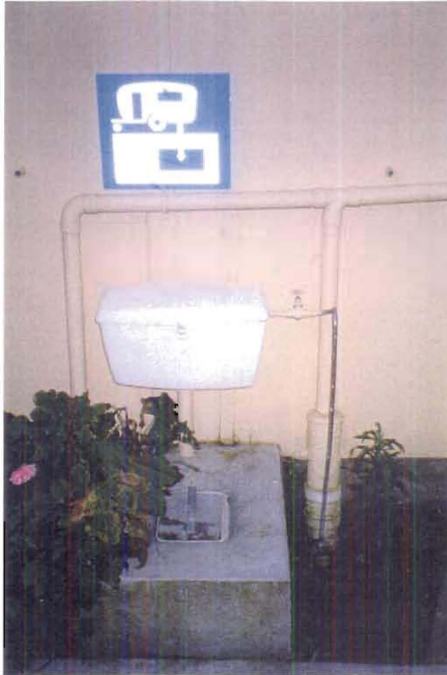
Plate 2. Effluent Disposal Facility In A Private Camping Ground.
