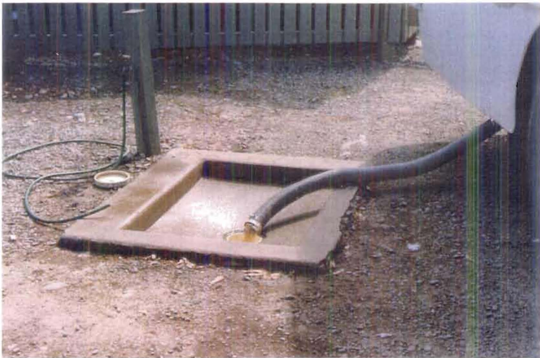
Plate 3. Effluent Disposal Facility Without Standard Fitting (Hose At Side For Washing Down).
