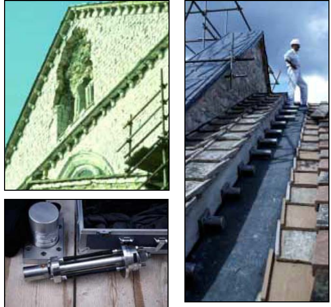
Figure 17. Basilica of S. Francis in Assisi: damage to the tympanum after the main earthquake event of September 26, 1997; retrofit intervention at the tympanum-roof connection with three groups of SMA devices (Croci et al, 2000)
