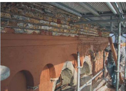
Figure 25. Transverse external post-tensioning for the retrofit of a masonry building
