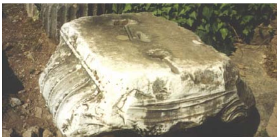
Figure 21. Typical use of rocking systems and segmental (multi-block) construction in the practice of ancient Greek and Roman Temples: axial load for re-centring; use of a lead element as shear and torsion key
