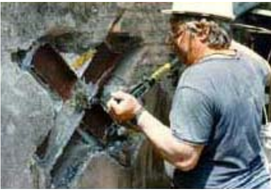
Figure 23. Manual post-tensioning of a post-tensioning “chain” for retrofit
