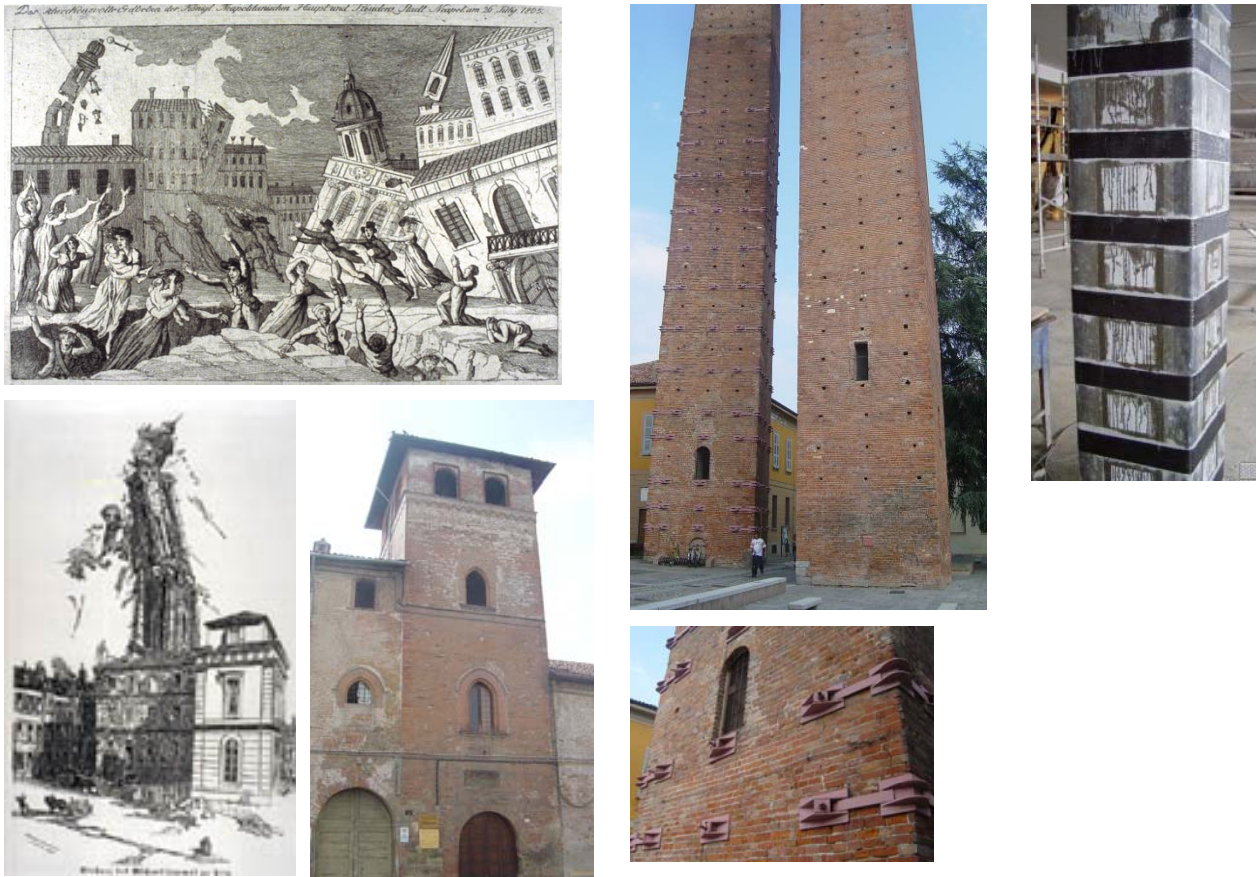
Figure 27. Left: typical representations of collapse of towers during historical seismic events (Napoli, 1806, Tuscany, 1896): awareness of their intrinsic vulnerability. Modern use of a half-collapsed medieval tower as a residential private house in Pavia, Italy Right: application of a temporary retrofit intervention based on transverse post-tensioning and confinement of the corners to a medieval tower in Pavia, after the collapse of the Cathedral Bell Tower in 1989. Far Right: Implementation of similar intervention by using FRP composite materials
