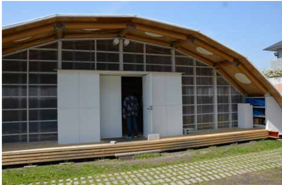
FIGURE 4.94 Shigeru Ban Studio at KUAD, front wall, 2013
