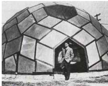
FIGURE 4.10 Dome shaped building by students of McGill University and Buckminster Fuller, Montreal, 1957
