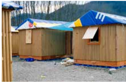
FIGURE 5.24 Paper Log House, Turkey, 2000
