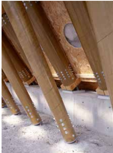
FIGURE 4.42 Paper Dome – connection with the foundation, 1998
