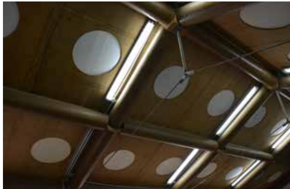
FIGURE 4.83 Hualin Primary School – roof structure, 2013
