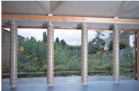
FIGURE 4.66 Westborough Primary School, paper tubes structure at the northern side of the building, 2001
