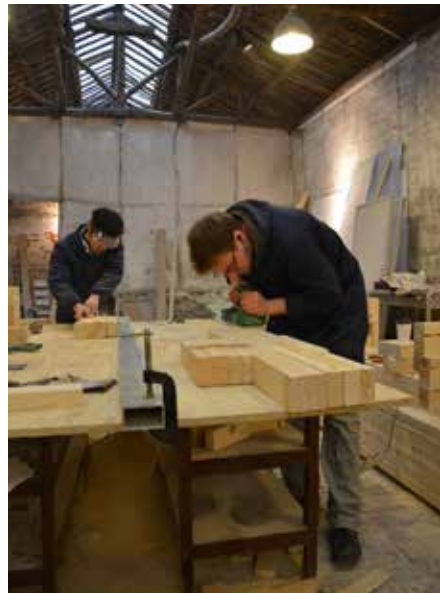
FIGURE 4.102 Miao Miao Paper Nursery School, preparation of wooden joints in Chengdu, 2013
