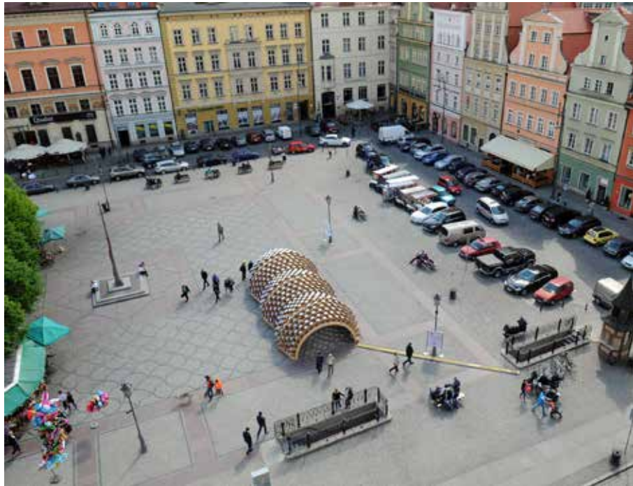
FIGURE 4.146 WUST Pavilion on Solny Square, Wroclaw, 2015
