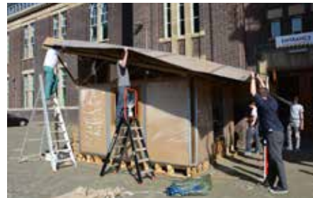
FIGURE 7.29 Construction of the roof
