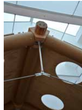
FIGURE 4.84 Hualin Primary School – 1:1 scale mock-up, roof structure, 2013
