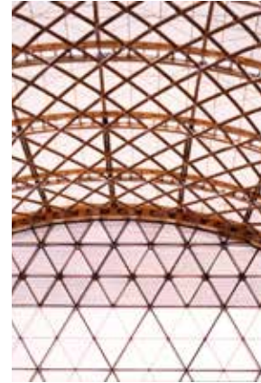
FIGURE 4.60 Detail of a gable wall, 2000
