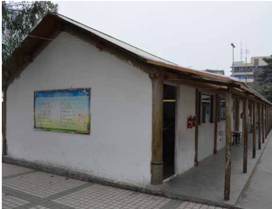
FIGURE 4.77 Hualin Primary School, Chengdu, China, 2013
