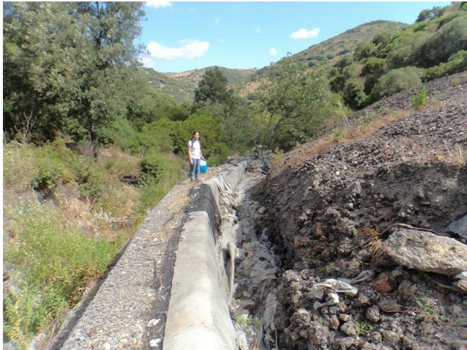
Figure 3.3 Erosion of slag waste after summer storms (date: 30.07.2014).
