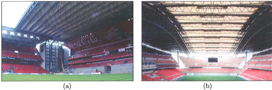
Figure 2.4: Folding membrane roofs at (a) Parken Stadium (Courtesy of CENO Tec), and (b) Toyota Stadium (Shibata, 2003)
