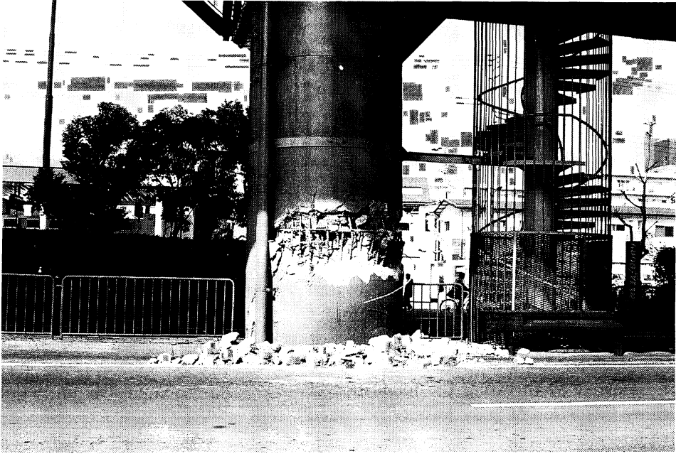
Photo. 2. Compressive failure mode due to impulsive force in a bridge R/C pier
