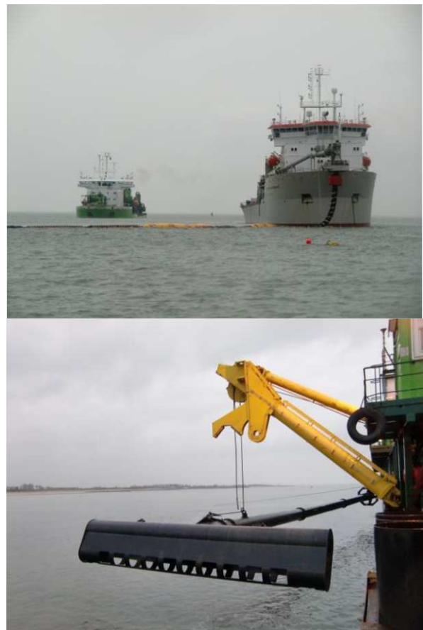
Figure 6. TSHD connected to floating line (above) and detail of diffuser head (below).
