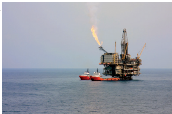
Figure 6.3. Offshore oil platform with support ships
