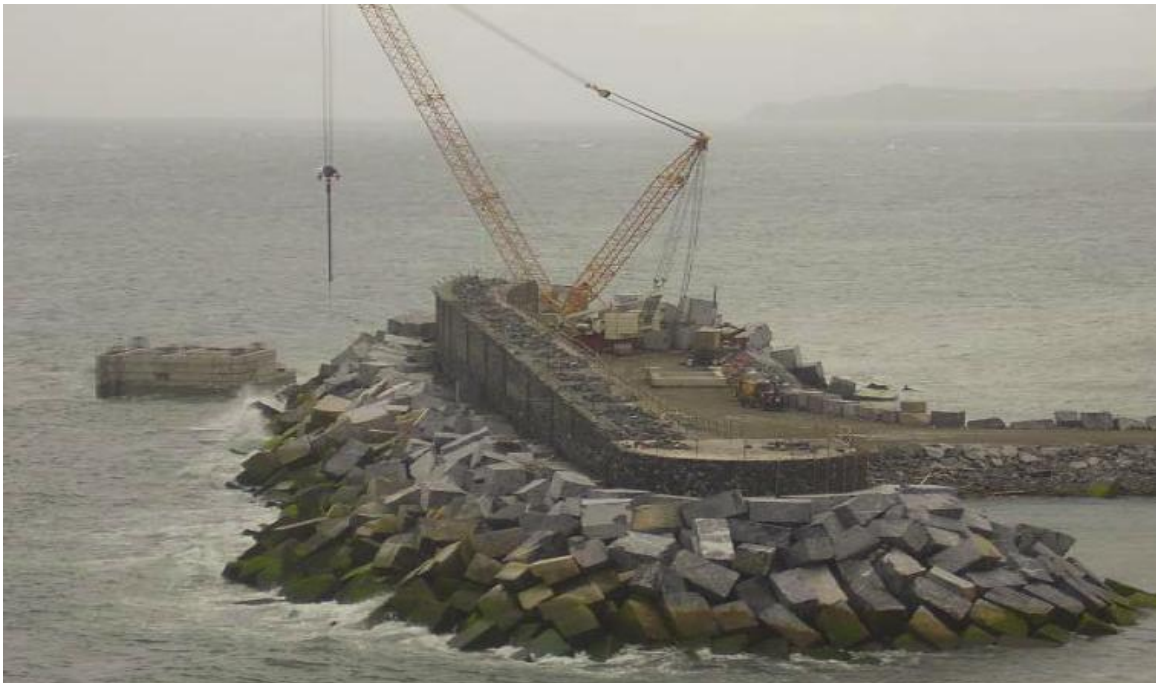
Figure 10: Construction of the Mutriku breakwater and air compression chambers (left).
