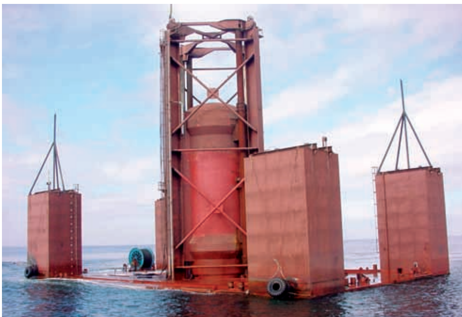
■ Archimedes Wave Swing: pilotproject met 2MW prototype (AWS ocean energy TLD)
