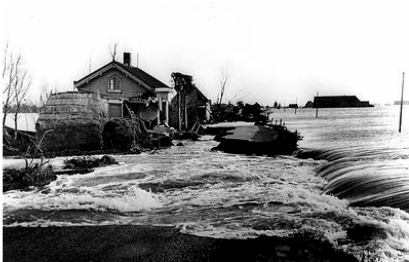
Figure 4 Dike breach during 1953 disaster
