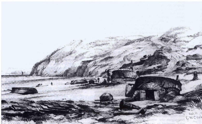
Fig. 2. Cellar settlement at Barepta, Cornwall County. (Courtesy of the Royal Institution of Cornwall)
