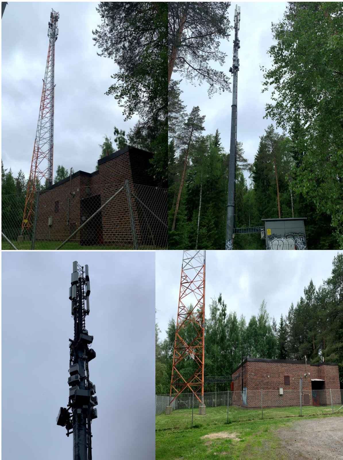
Figure 1 The field images of the deployed base station with GBT in regions of Finland.
