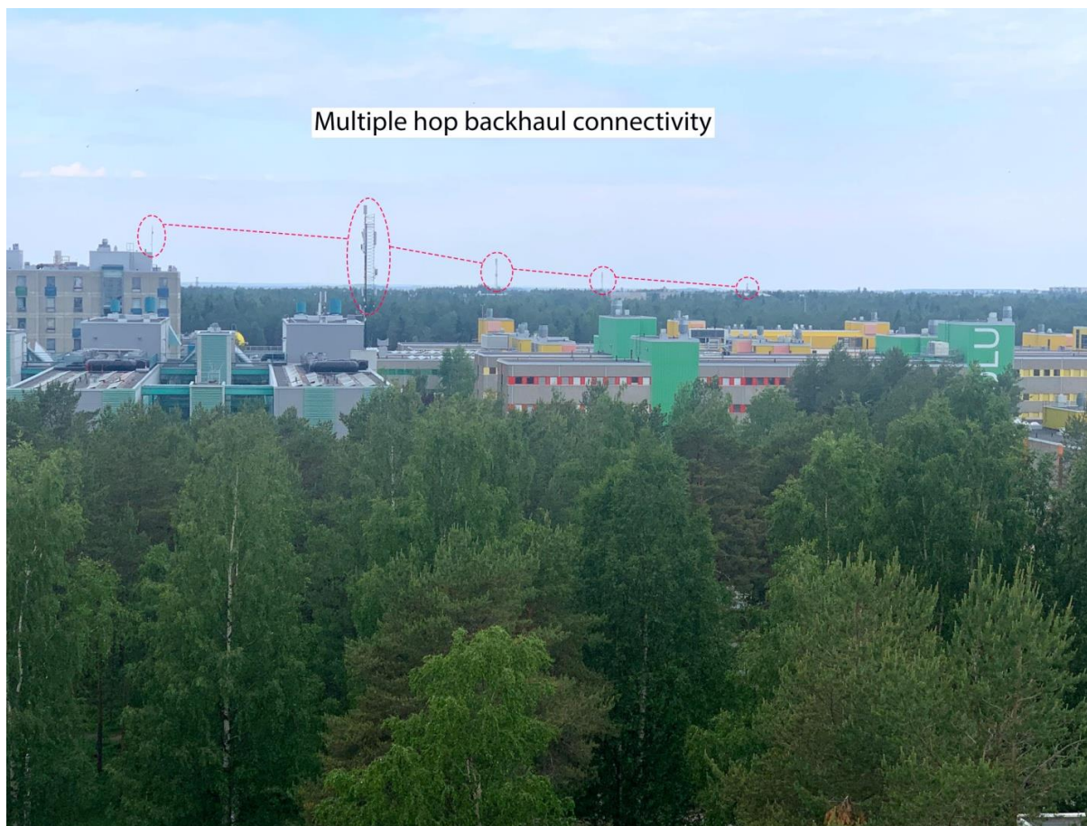
Figure 4 Possibilities of backhauling connectivity with multiple hops.
