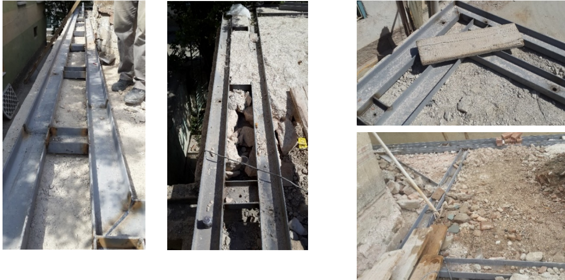
Fig. 8. Application of double steel girder (2U160) on the load-bearing walls
