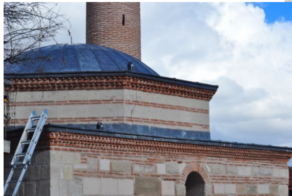
Fig. 9. Lead covering after steel girder retrofitting
