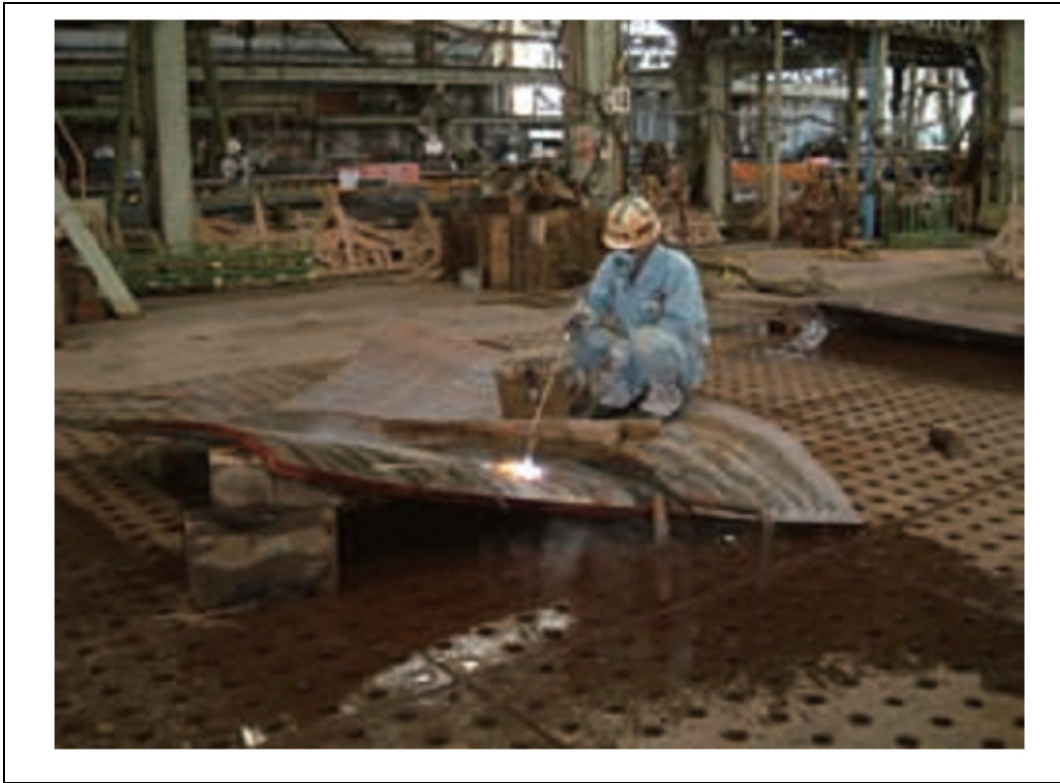
Figure 2.10 Example of conventional line heating work (Yoshihiko et al. , 2011)
