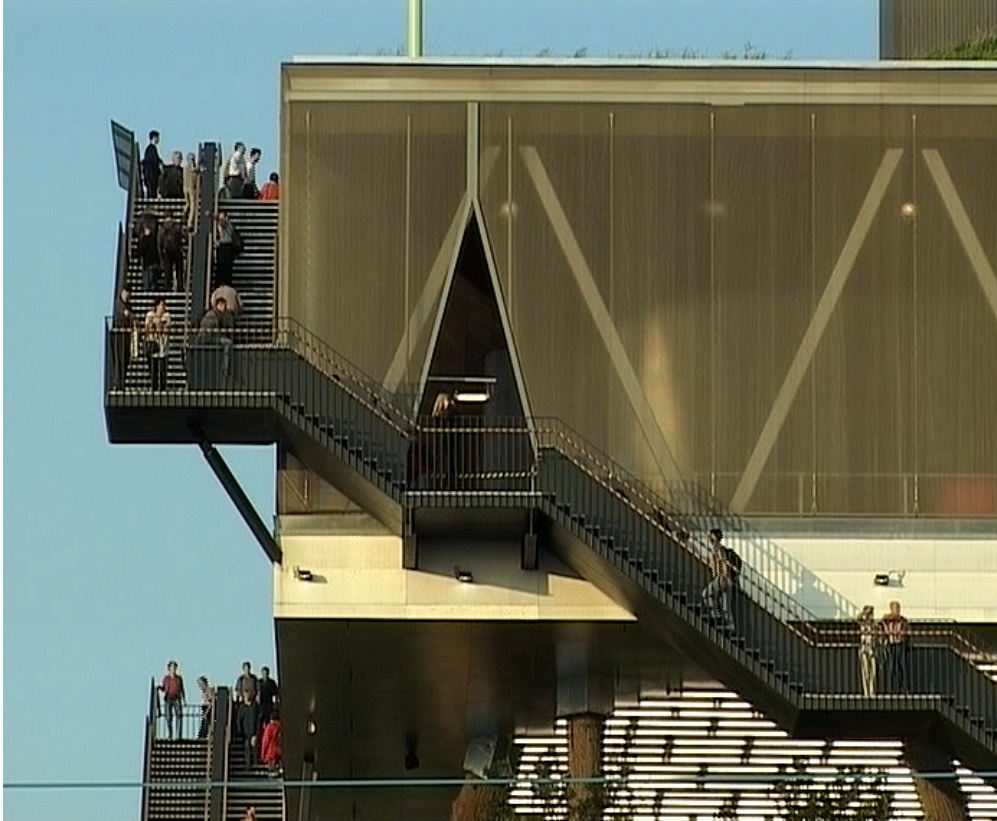
Figure 4.6: The walking times were measured at the part of the 18 stairs at the right to the triangle-shaped door (platform to platform). The whole stairway had this design of an alternation of stairs and platforms.
