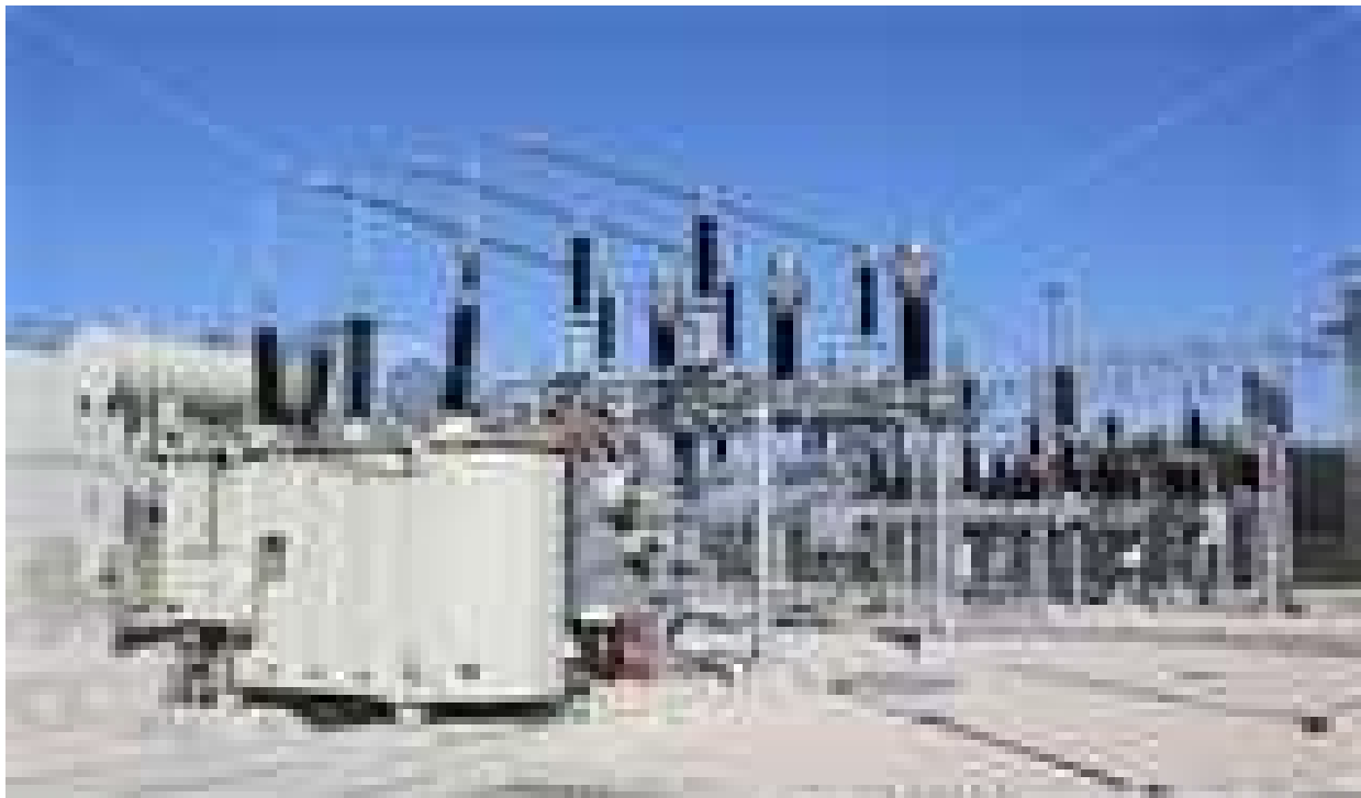
Fig 2.2: Distribution Transformer
