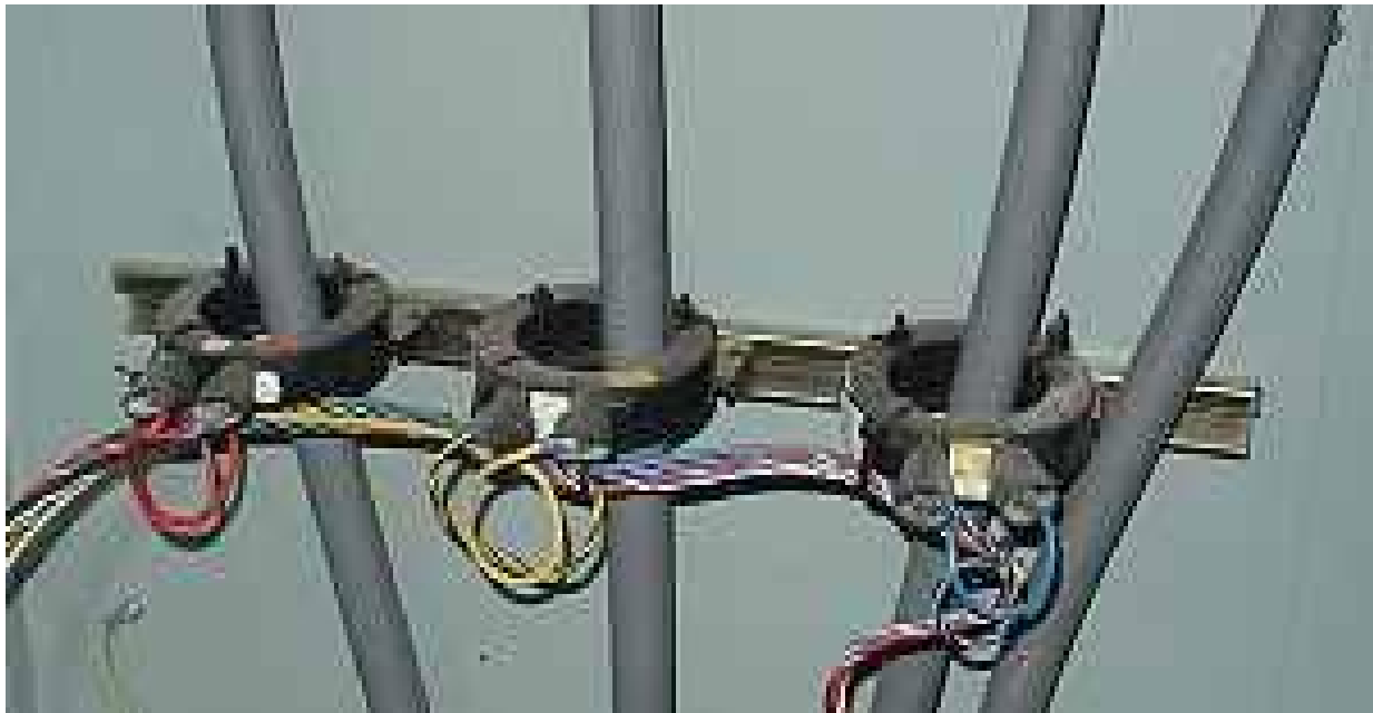
Fig 2.3: Current Transformers.
