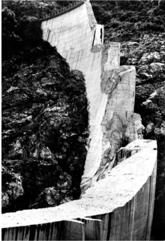
Figure 2: The remains of the Malpasset dam
