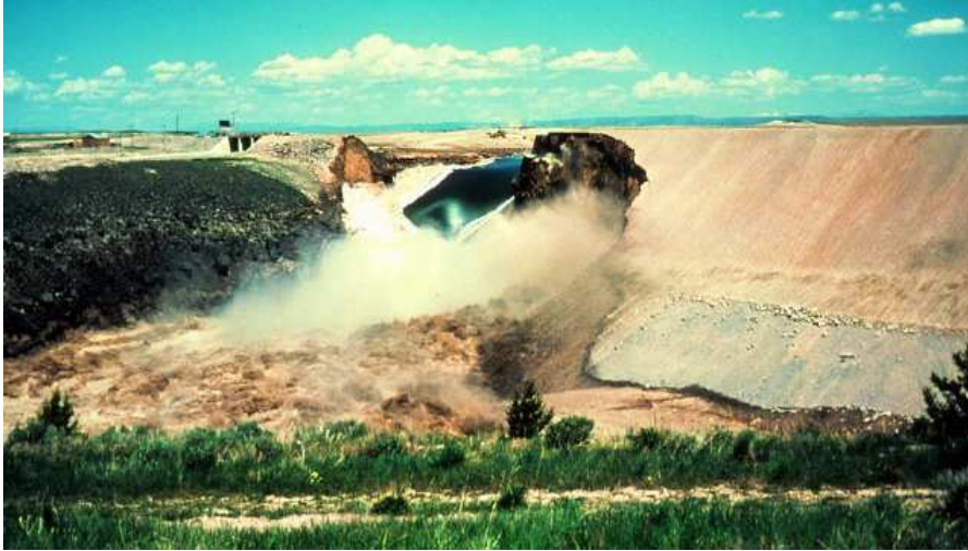
Figure 1: The teton dam shortly after breach
