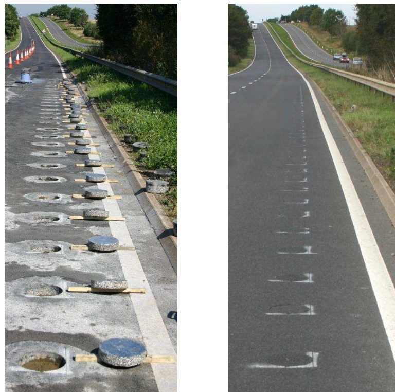
Figure 5.1 Asphalt discs in lane 2 of the A5 sites, about to be installed (left) and shortly after installation (right)
