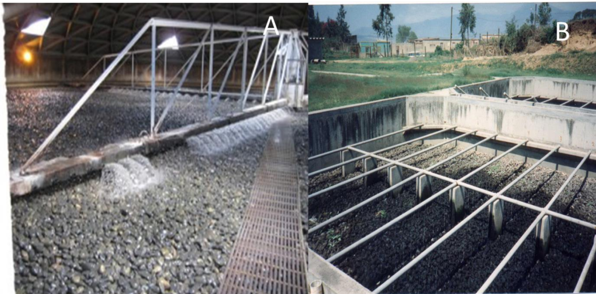
Figure 4.3: A) Large-scale indoor rock filtration unit for the treatment of wastewater, City of Yakima, Washington, USA. B) Static trickling filter with wastewater being dispersed over volcanic rock media, using gravity flow in the Republic of Guatemala. URL: http://www.yakimawa.gov/ and URL: http://www.cep.unep.org
