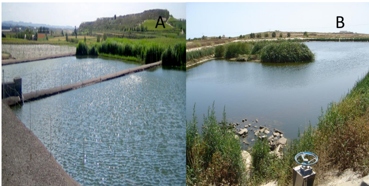
Figure 4.1: A) Maturation Ponds in series, designed by the Department of Hydraulics, Maritime and Environmental Engineering (DEHMA)© UPC, in Verdú - Lleida, Spain. B) Maturation Pond as a tertiary treatment unit in Korba, Tunisia. URL: http://athene.geo.univie.ac.at/pucher/gallery/view_album.php and URL: http://gemma.upc.edu/
