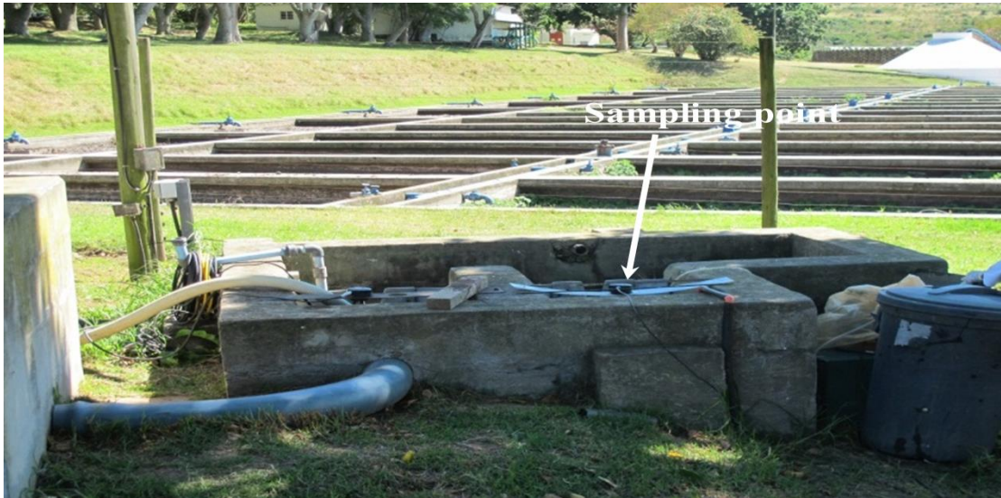
Figure 1.2: SB from the IAPS final effluent. From here the effluent flows into the different tertiary treatment systems: Maturation Pond; Slow Sand Filter; Rock Filter.
