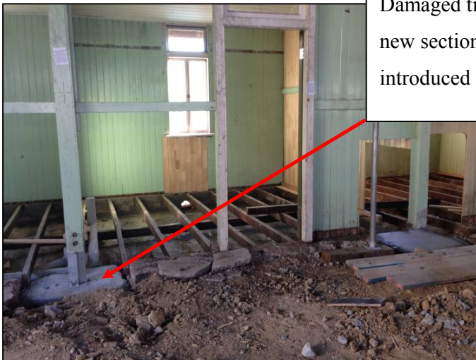
New footing and slab
