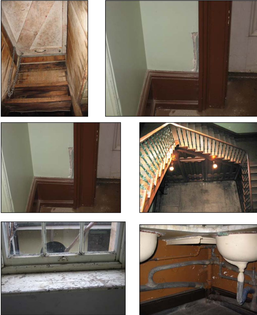
Figure 5.6: Photo-documentation of the building condition - interior 2
