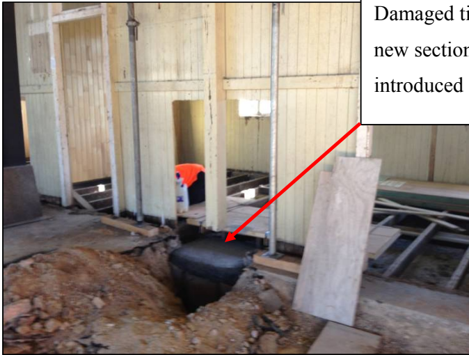
Damaged timber columns cut and new sections/splicing detail introduced as well as new footing
