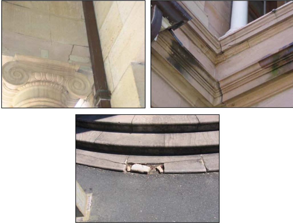
Figure 5.5: Photo-documentation of the building condition- exterior 1
