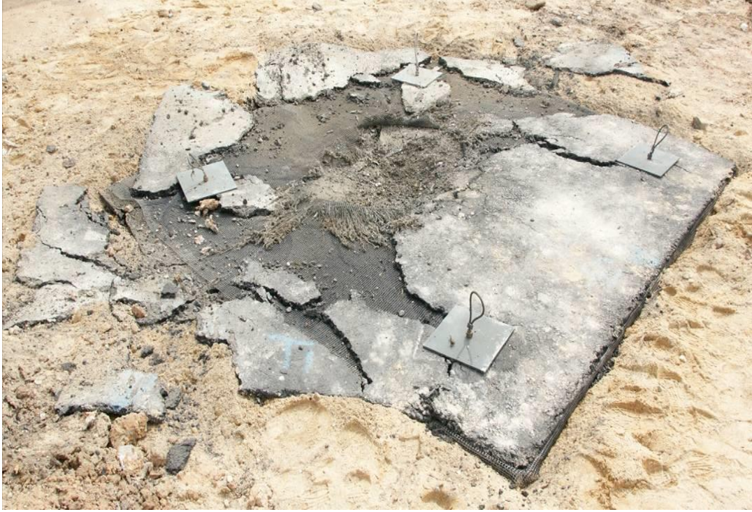
Figure 19. Damage of the multi-layer pavement after blast load with top layer AC in place
