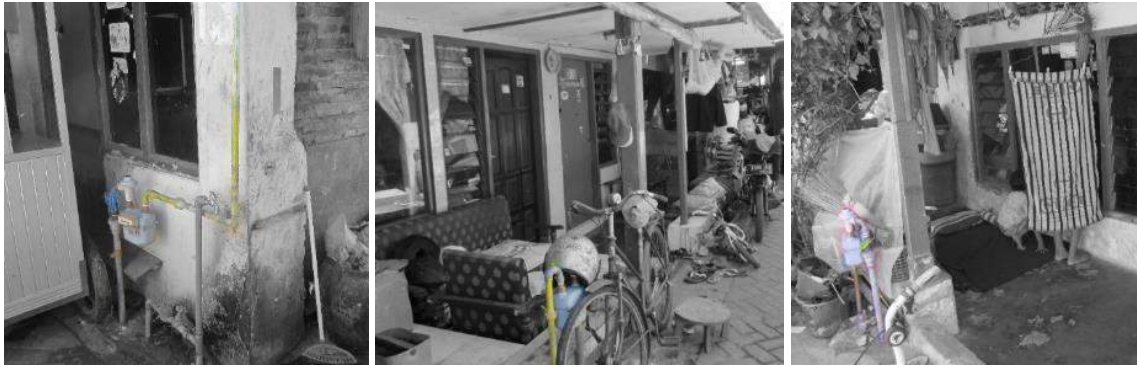
Figure 5.25 Natural gas pipes (highlighted in colour) for individual houses in Rungkut Lor
